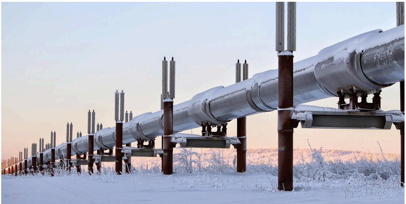
The Trans Alaska Pipeline transports oil from Alaska's north slope to ports on the Gulf of Alaska for shipping. Photo by Robzor, Pixabay , licensed under Pixabay .
