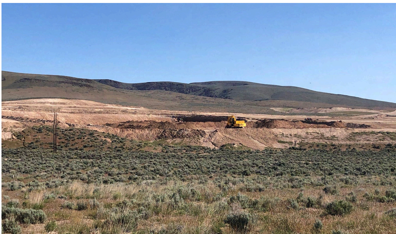
Thacker Pass Lithium Mine under construction in 2024. Photo by Emmett Hopkins.
